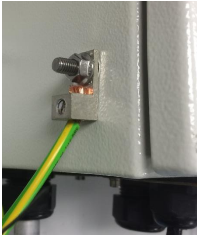
Figure 5-25: Position of primary protective earth bonding lug
